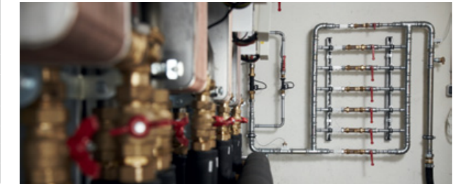
Hydraulic "harp" to regulate draw-off volumes
